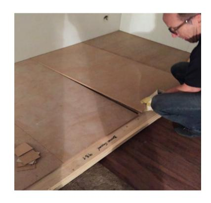
The floor parts are clearly marked. Some customers use to fill the space between floor and Booth with regular Rockwool.
