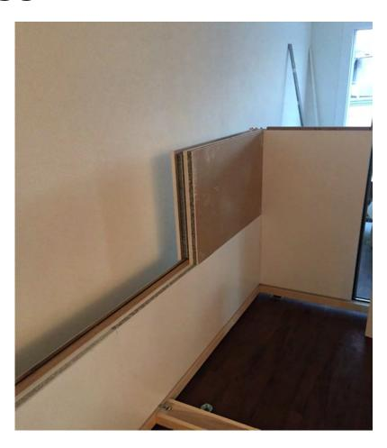
Move the bricks parallel with a rubber hammer. A White rubber hammer will do. Try to position the door and window parts with an inclination (like a sicar)
