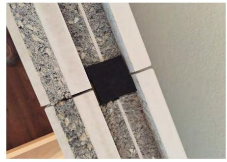
In a regular Project there are 4 levels of Bricks. Level A, B and C all 60 cm (approx 2 ft) and level D 30 cm (approx 1 ft). Between every level comes this kind of stick, In this case between Level C and D.
